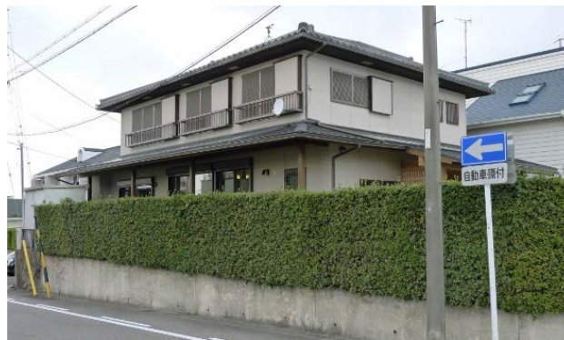
Figure 5. Outside view of House N after renovation.
